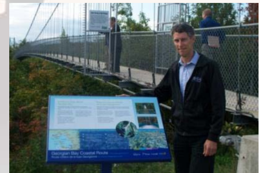
Scenic Caves Suspension Bridge
