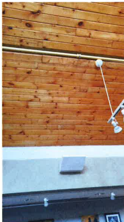
Photograph 4: Example of past wood staining on underside of wood planks
