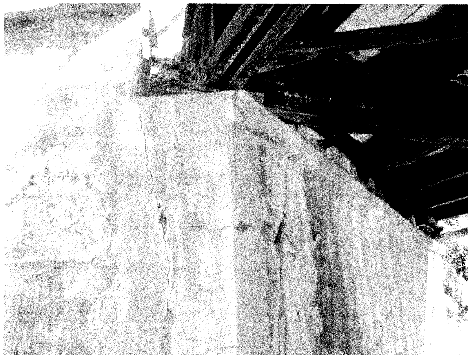
North West Corner
