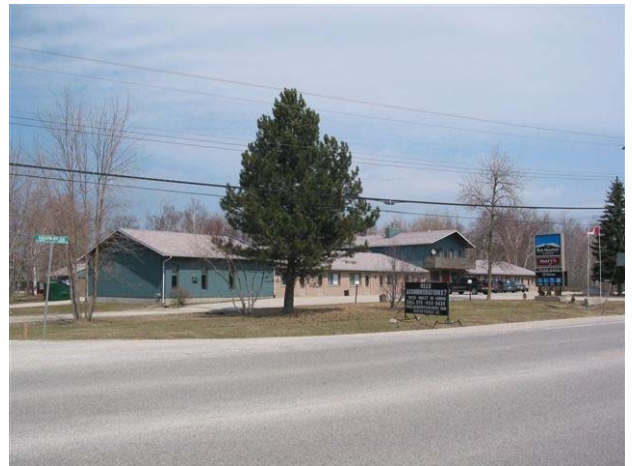
Plate 2. Disturbed Lands, Southern Edge of Property (view north east)
