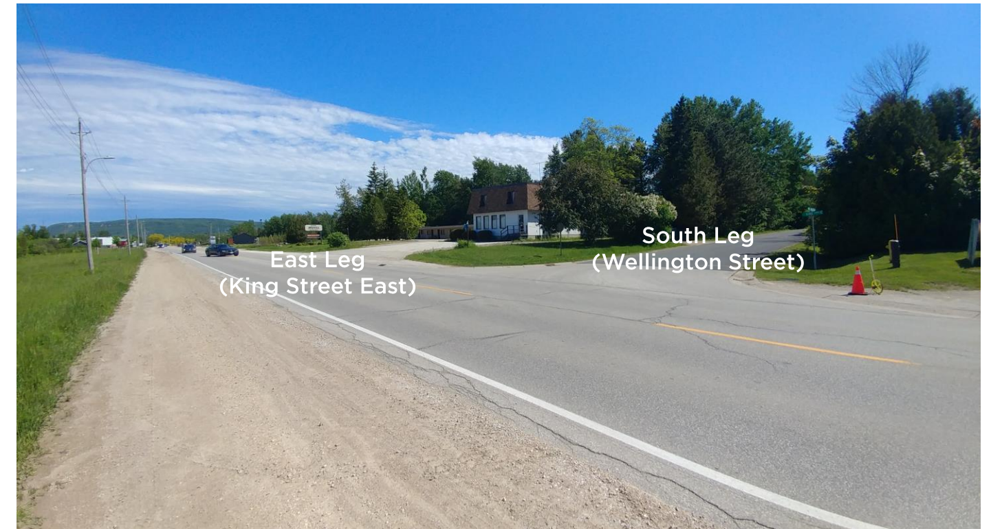
Intersection of King Street East & Wellington Street – south and east legs
