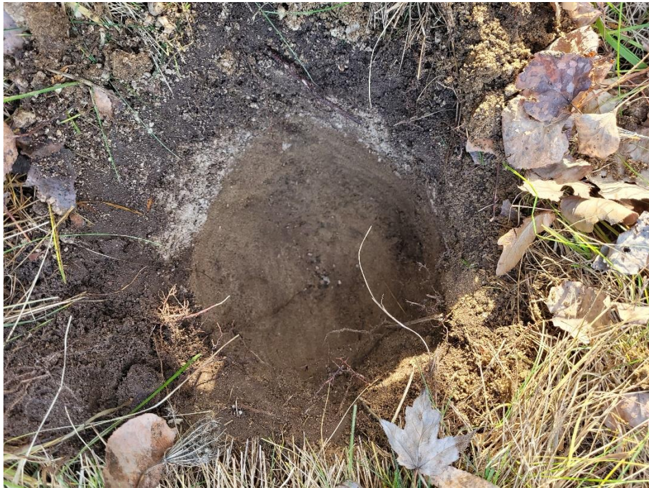
Image 12: Open Test Pit showing Subsurface Stratigraphy.
