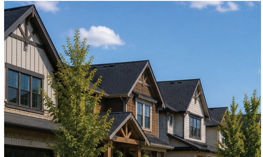
Example of varying roof forms within the streetscape
