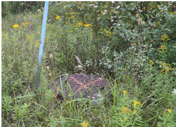
Figure 3. Existing maintenance holes.
