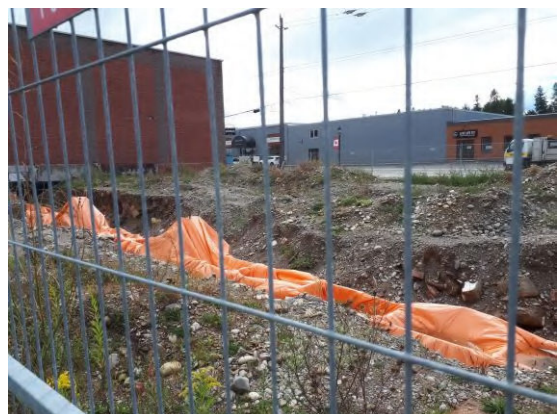
Picture 4: View of excavated material at the adjacent property to the south of the site.
