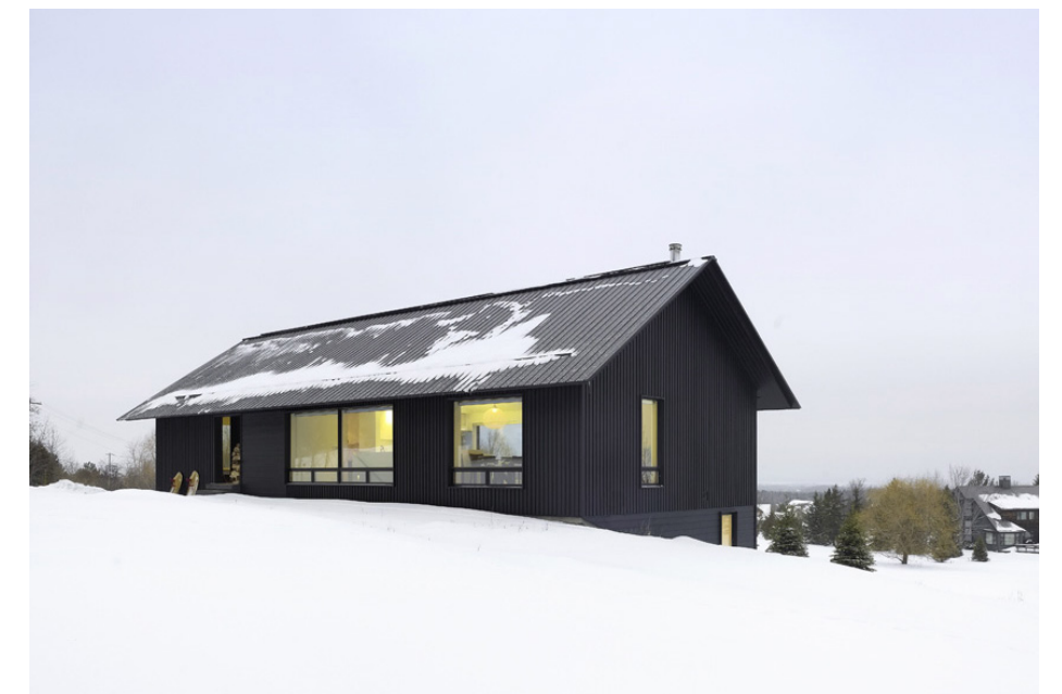
Clearview Chalet by Atelier Kastelic Buffey Clearview Township, Ontario
