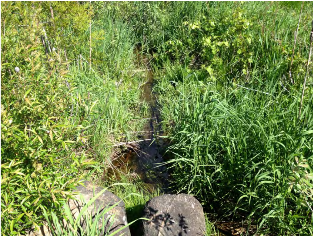
Photo No. 8: Portion of watercourse to be realigned, June 2017 flows
