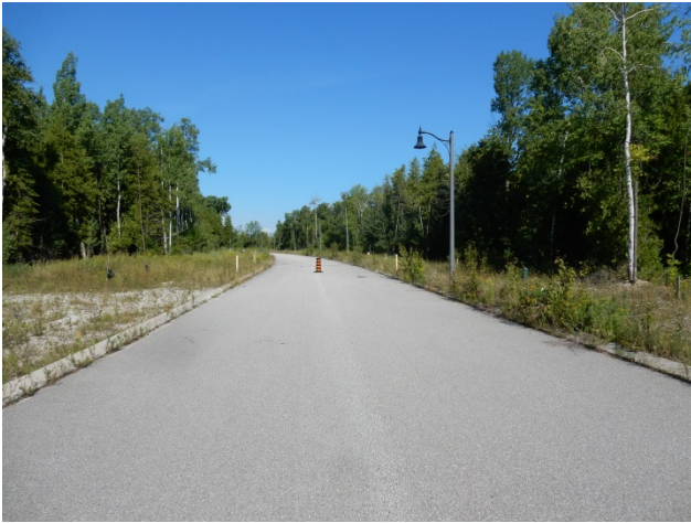
Image 5: View along roadway.
