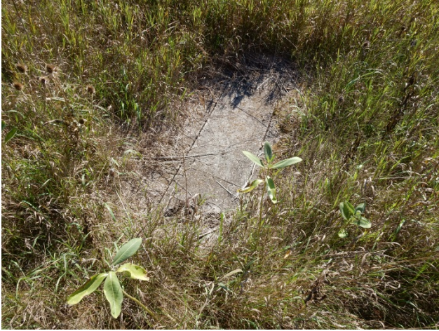
Image 13: Concrete hatch located in artificial plateau.
