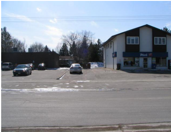
Uses along Highway No. 26 outside of the core in the Thornbury Commercial Area are generally oriented to passing motorists.
