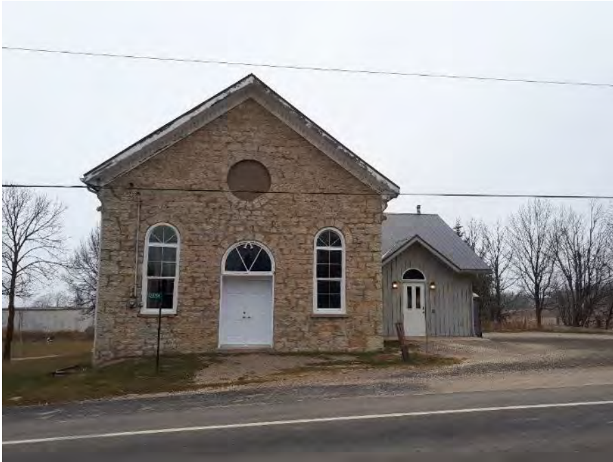
Image 13: Stone church in Ravenna, facing north.
