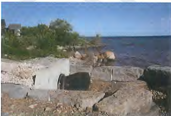
Photograph 7: Stormwater drainage culvert at Delphi Point in east Section of ANSI.
