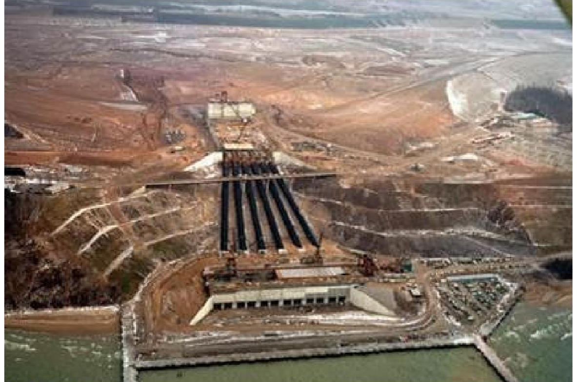
Construction of the Penstocks (turbines) at Ludington MI Site
