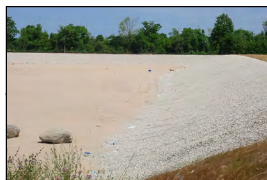
LINED PORTION OF LANDFILL
