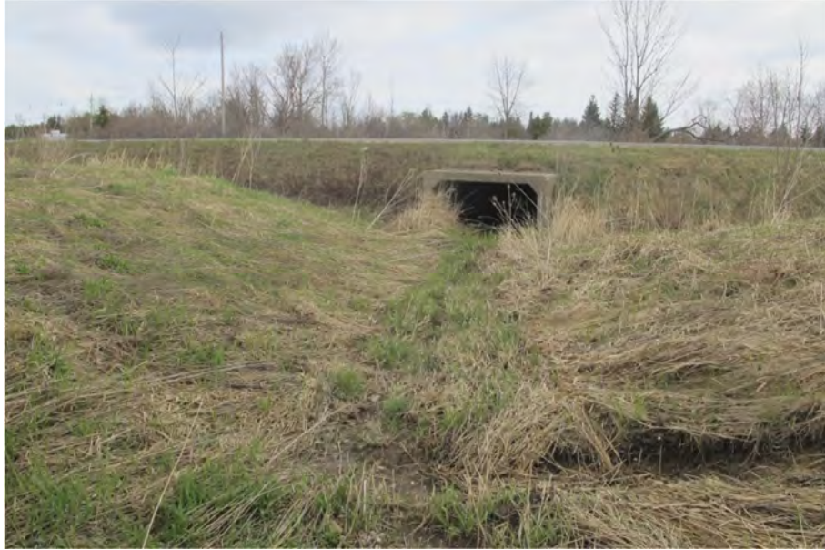
Photo – Concrete Box Culvert at Hwy 26 – Looking North (Nov. 2022)
