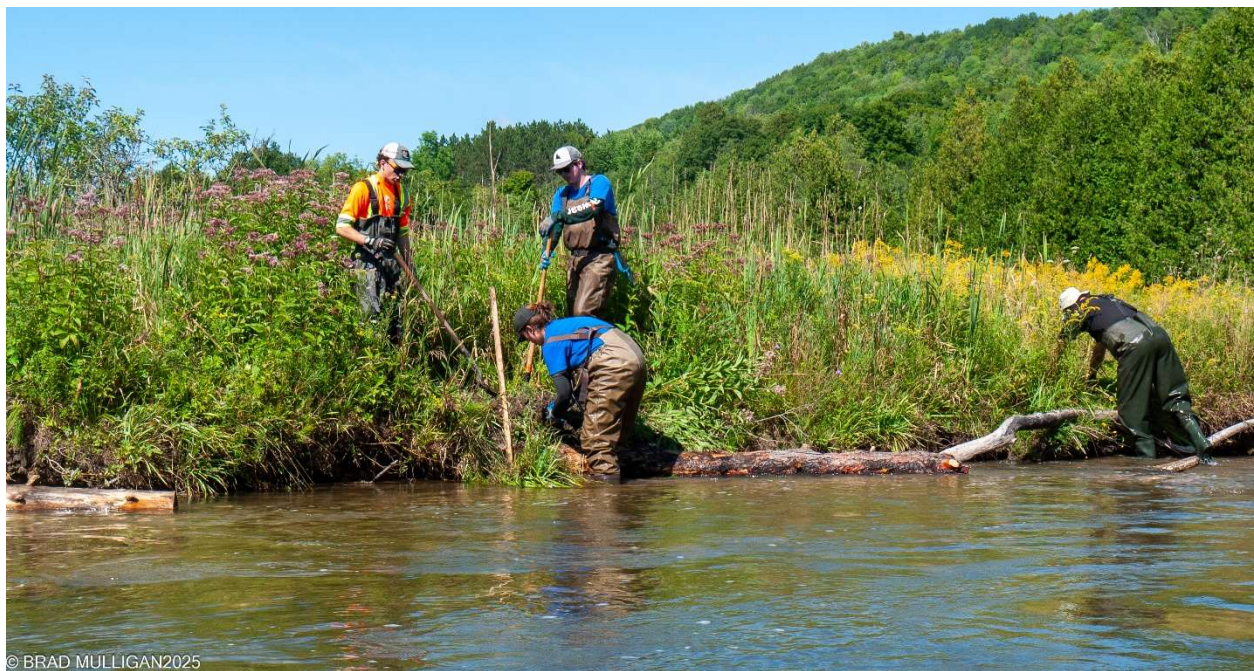
Installation of log deflectors
