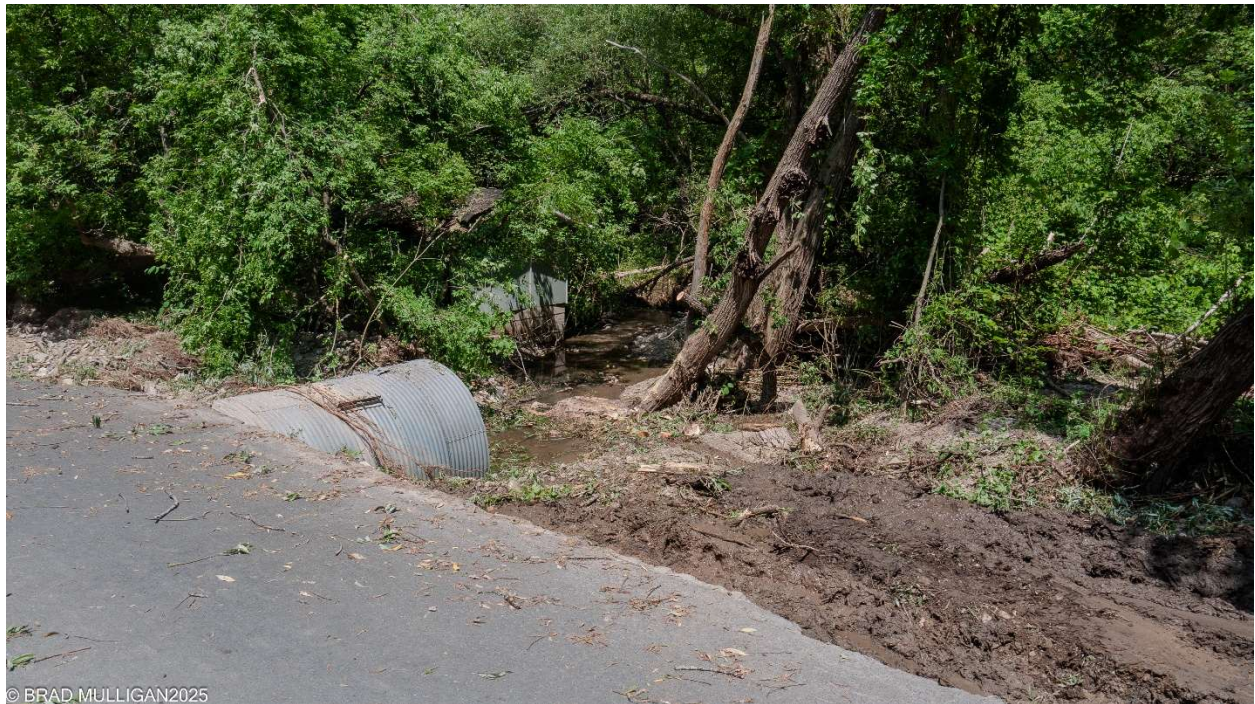
After removal – should help with flooding damage in future
