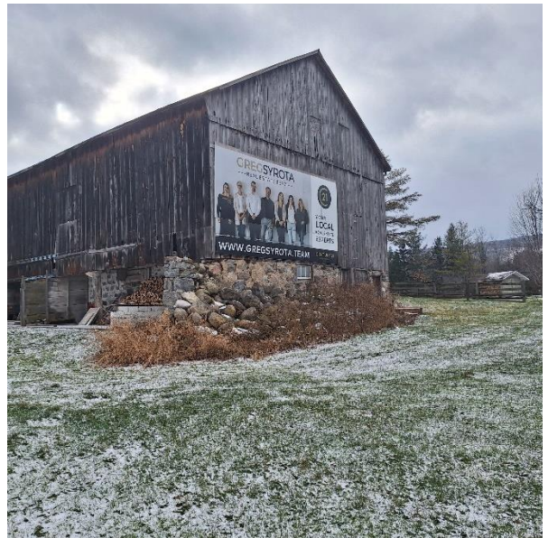
Image 4: Barn, facing southwest.
