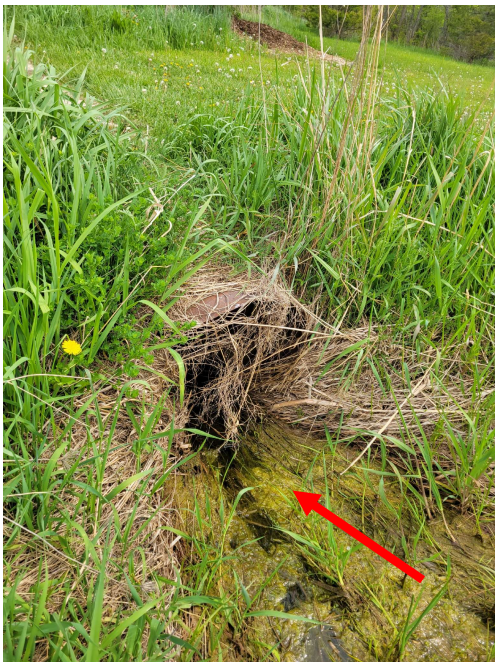
Photograph 6. Drainage feature crossing, upstream of CSP culvert (May 2023).
