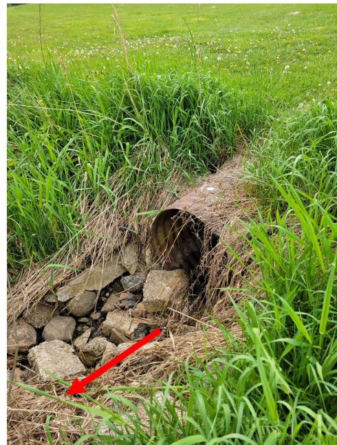
Photograph 7. Drainage feature crossing, downstream of CSP culvert (May 2023).
