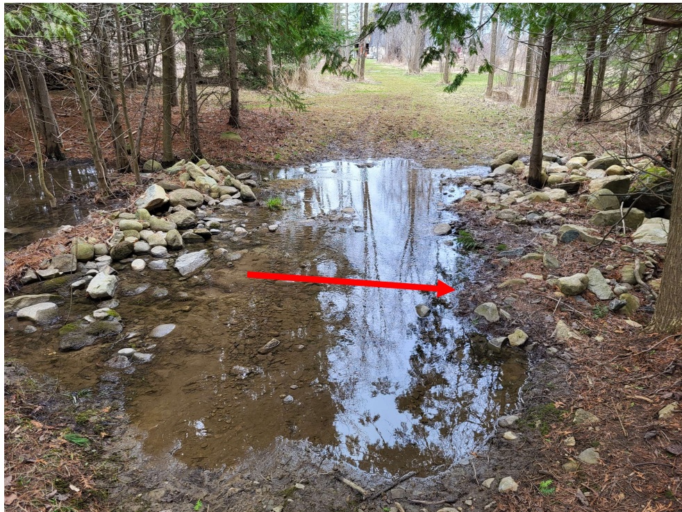
Photograph 2. Drainage feature crossing, creating a barrier to fish, looking north. (April 2024)
