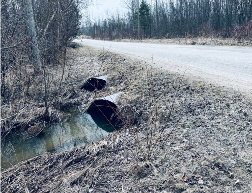
Photo #4 Double Culvert Crossing
