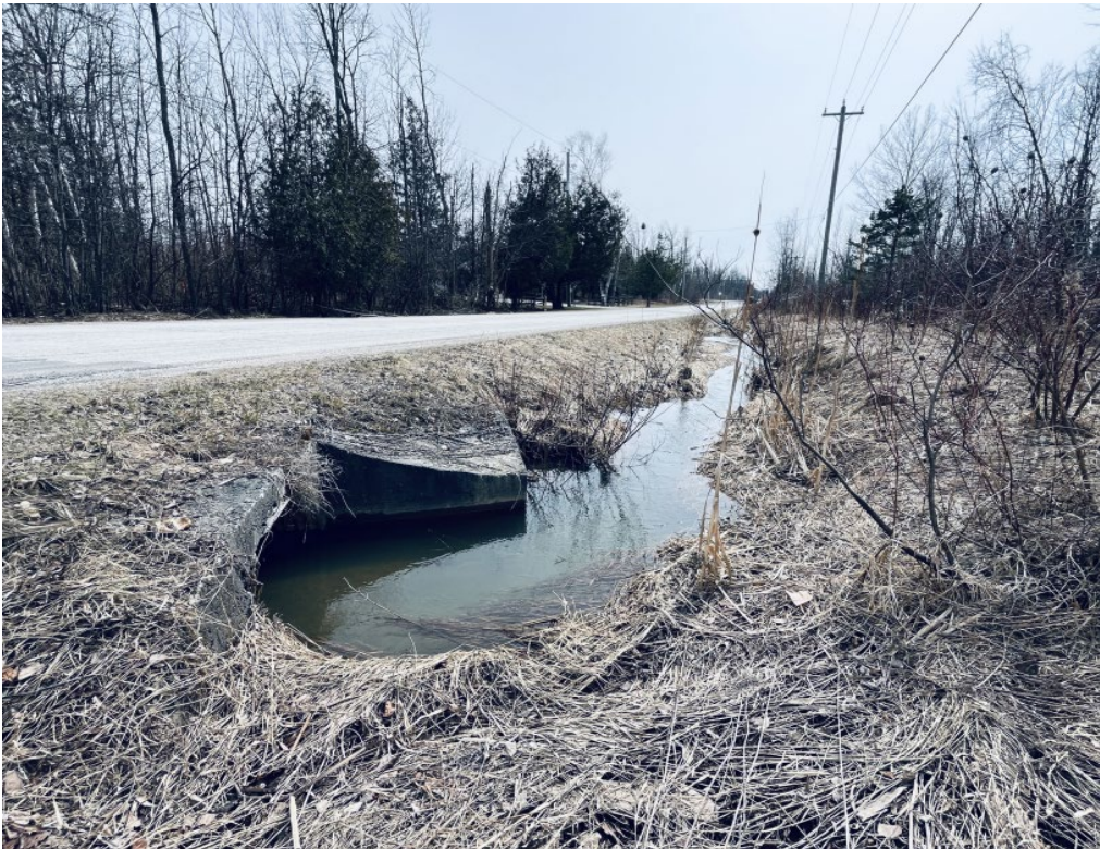
Photo #4 Double Culvert Crossing
