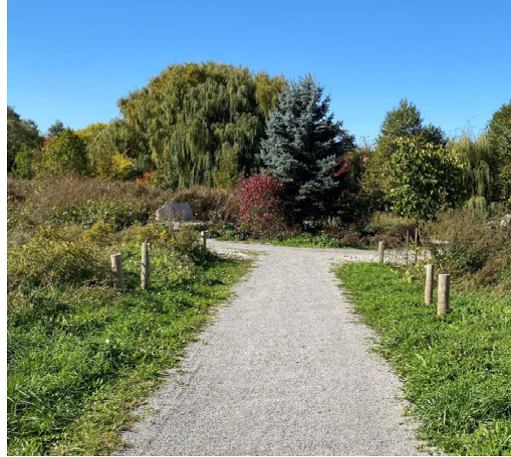
Compacted Stone Dust Pedestrian Path
