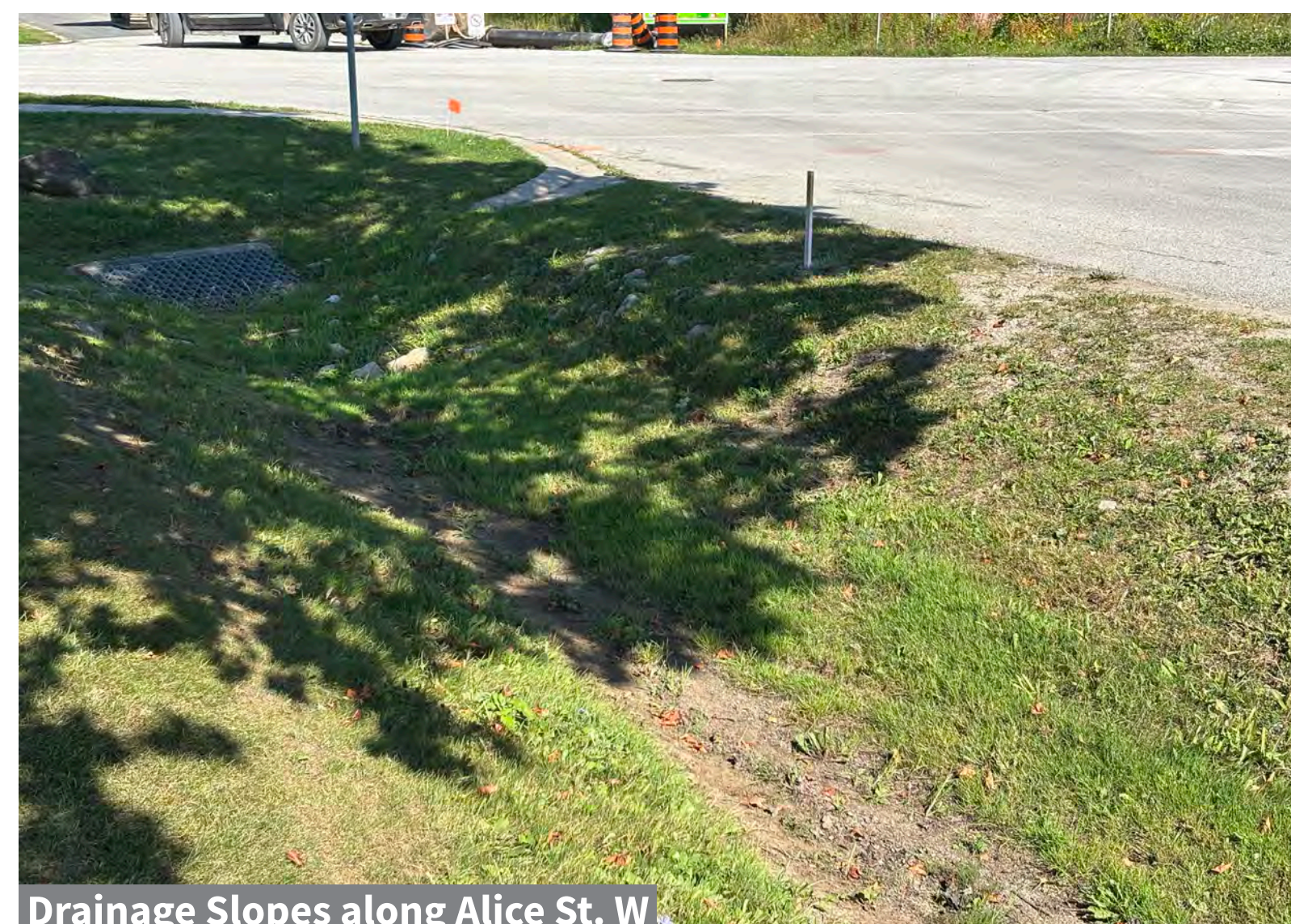
Drainage Slopes along Alice St. W
