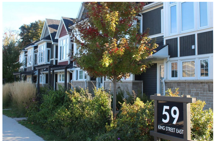
Locate townhouse blocks close to the property line with their primary façade and/or entrance addressing the street
