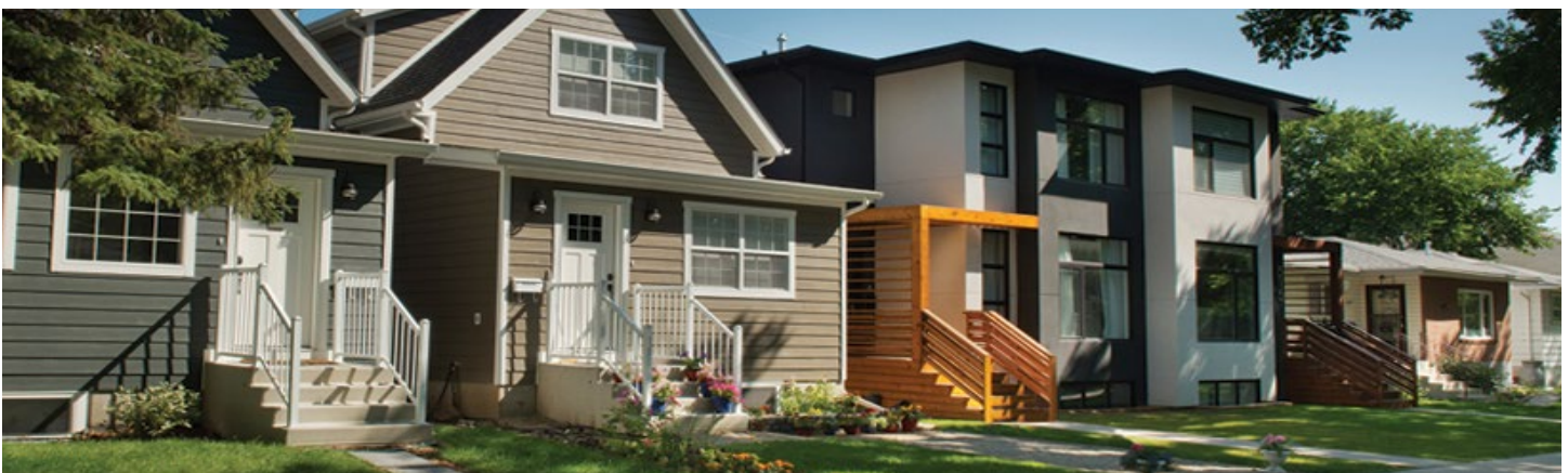
Maintain predominant front and side yard setbacks to preserve the existing rhythm of the street
