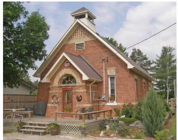
Repair or replace windows and doors with in-kind materials as key defining architectural elements
