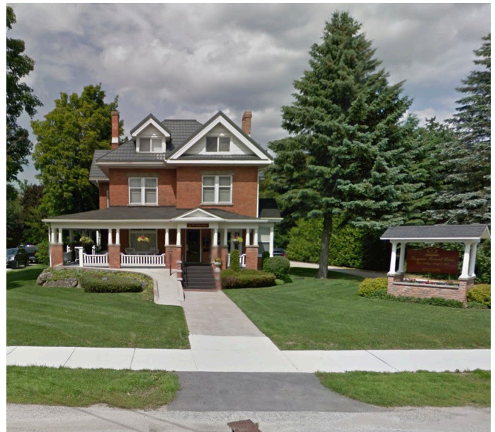
Converted dwelling in Thornbury
