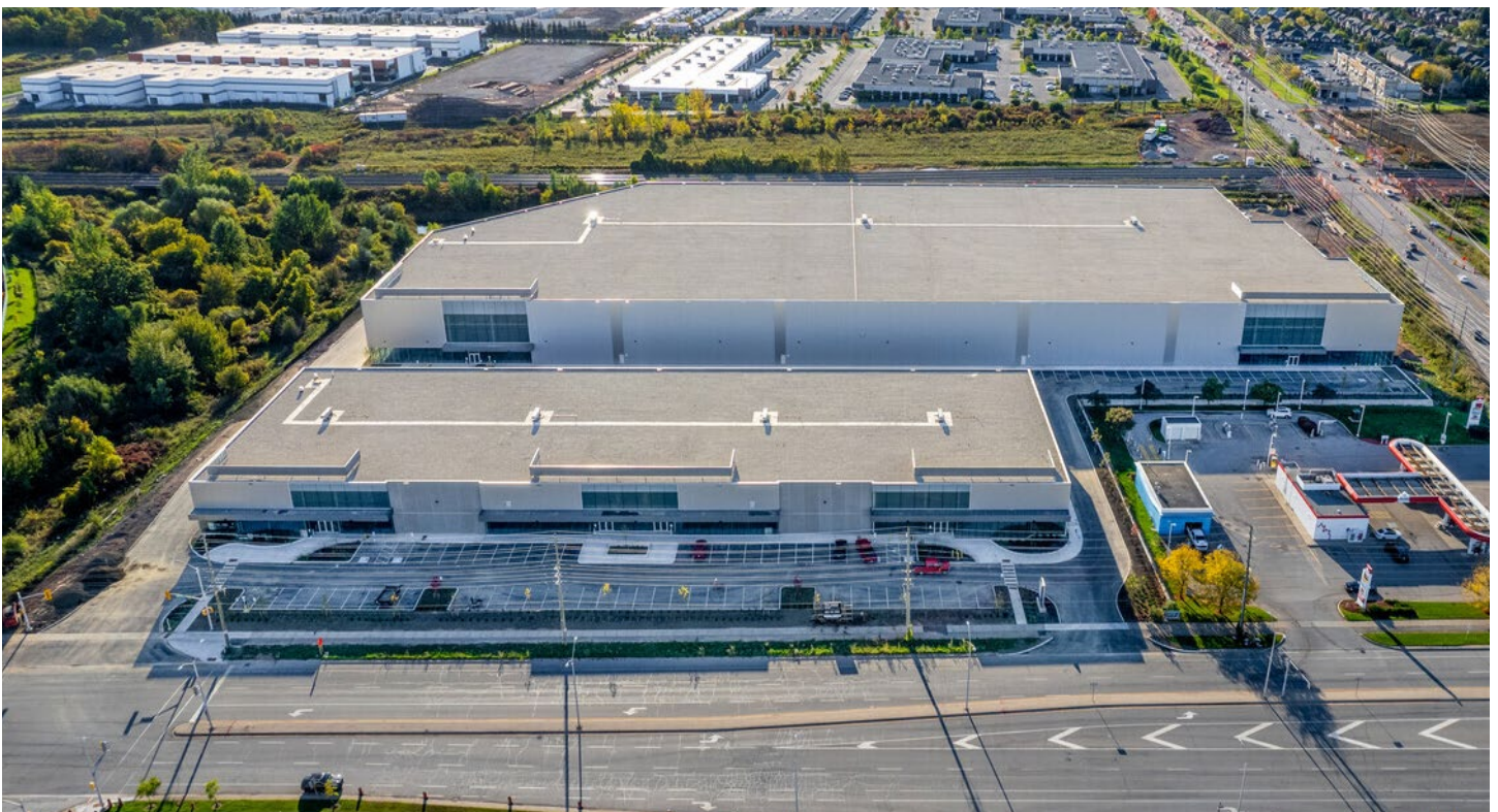
Site buildings close to the street edge and ensure main parking and industrial areas are located to the rear
