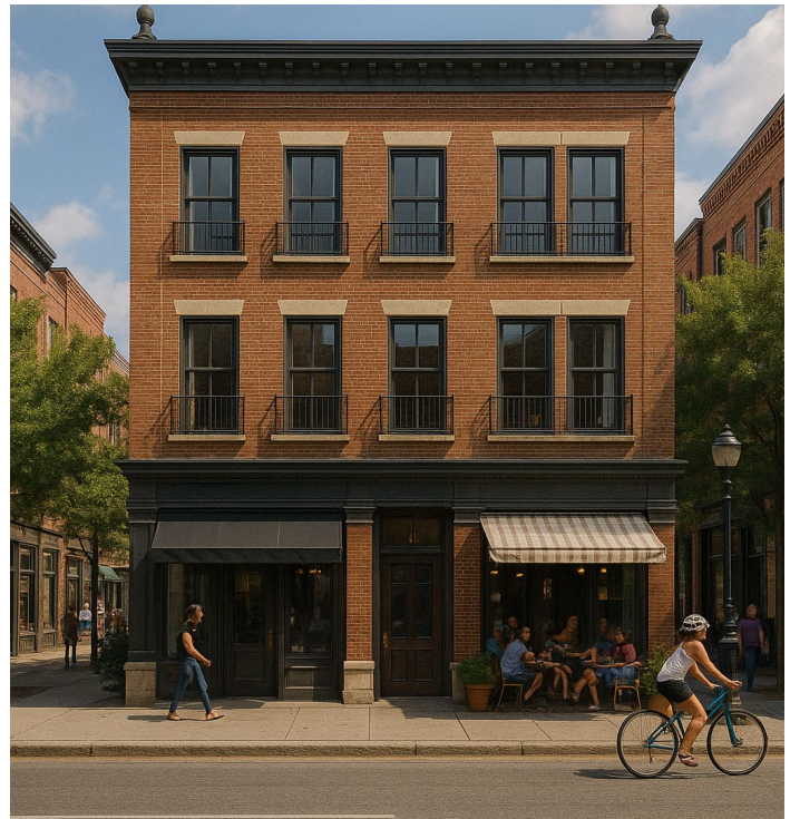
Provide a combination of horizontal elements such as sign bands, cornices, and projections and vertical elements such as changes in material, building articulation and columns
