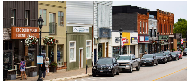
In Downtown Thornbury/Clarksburg, set back new buildings to align with the established streetwall and maintain a maximum three storey height
