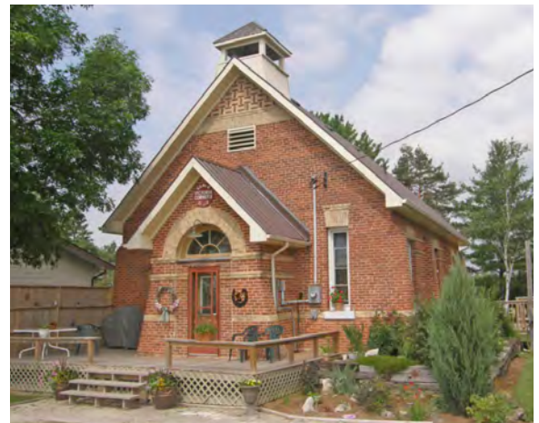
Repair or replace windows and doors with in-kind materials as key defining architectural elements
