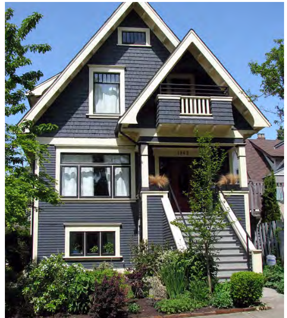
Exterior cladding materials should simulate the form, colour and profile of original materials
