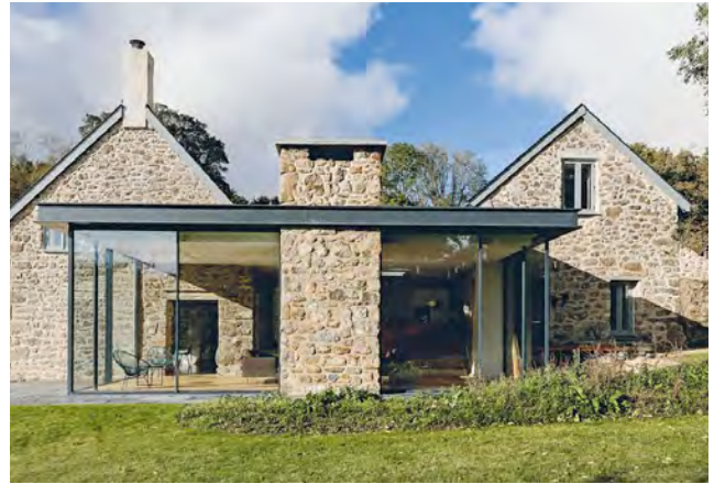
New design elements should be sympathetic and respectful towards the original structure
