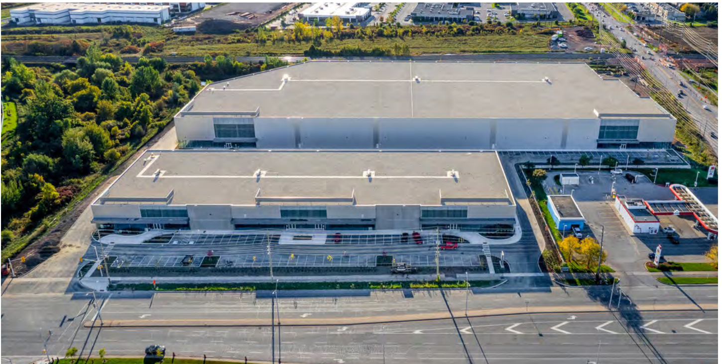
Site buildings close to the street edge and ensure main parking and industrial areas are located to the rear
