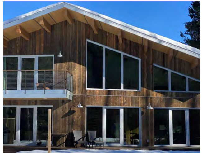
Large windows, roof overhangs and building orientation help support passive solar gain, natural daylighting and seasonal shading while contributing to year-round residential comfort.
