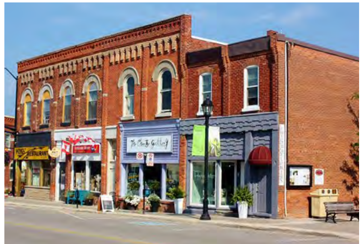
Divide larger facades through a symmetrical pattern of bays to emphasize individual units and single store facades
