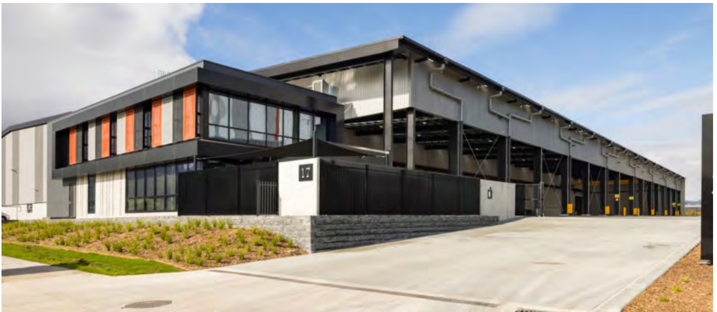
Orient loading bays and service areas to the side or rear of buildings
