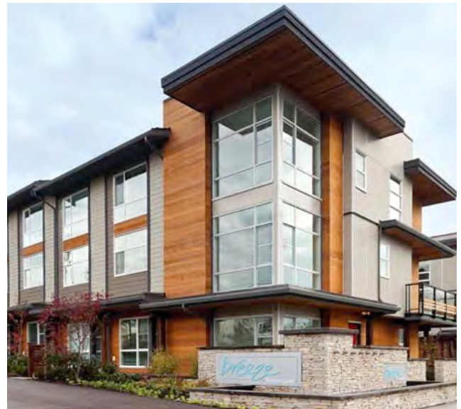
Roof overhangs and recessed upper-storey glazing help provide shade, weather protection and passive solar control while complementing architectural character.
