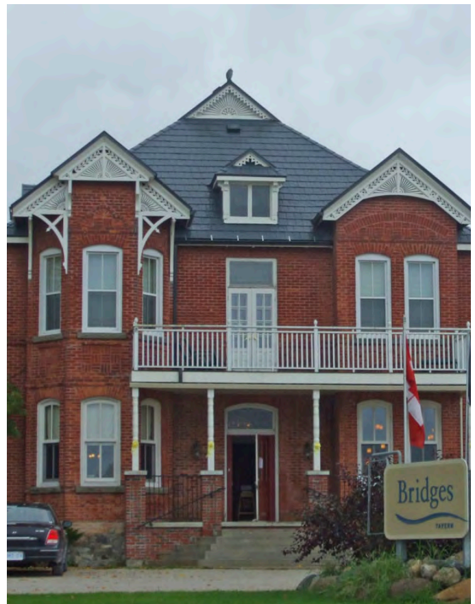
Restore roofing with materials consistent to the historic architectural style
