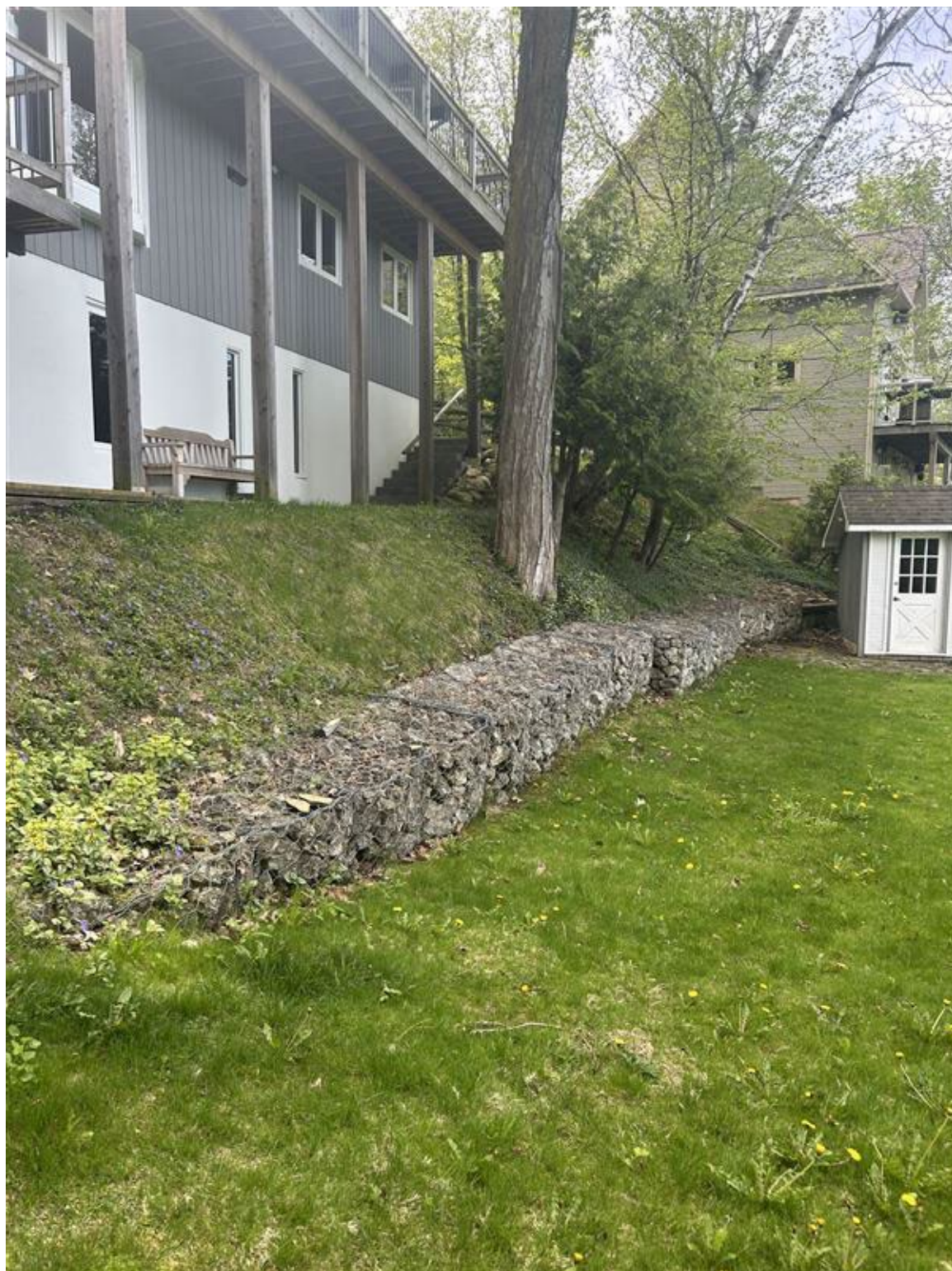
Photograph 4 – View of gabion basket retaining wall looking west
