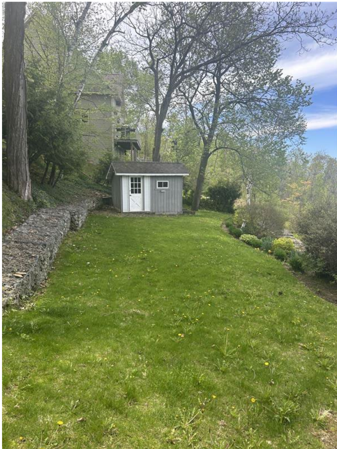
Photograph 8 – View of existing shed looking west
