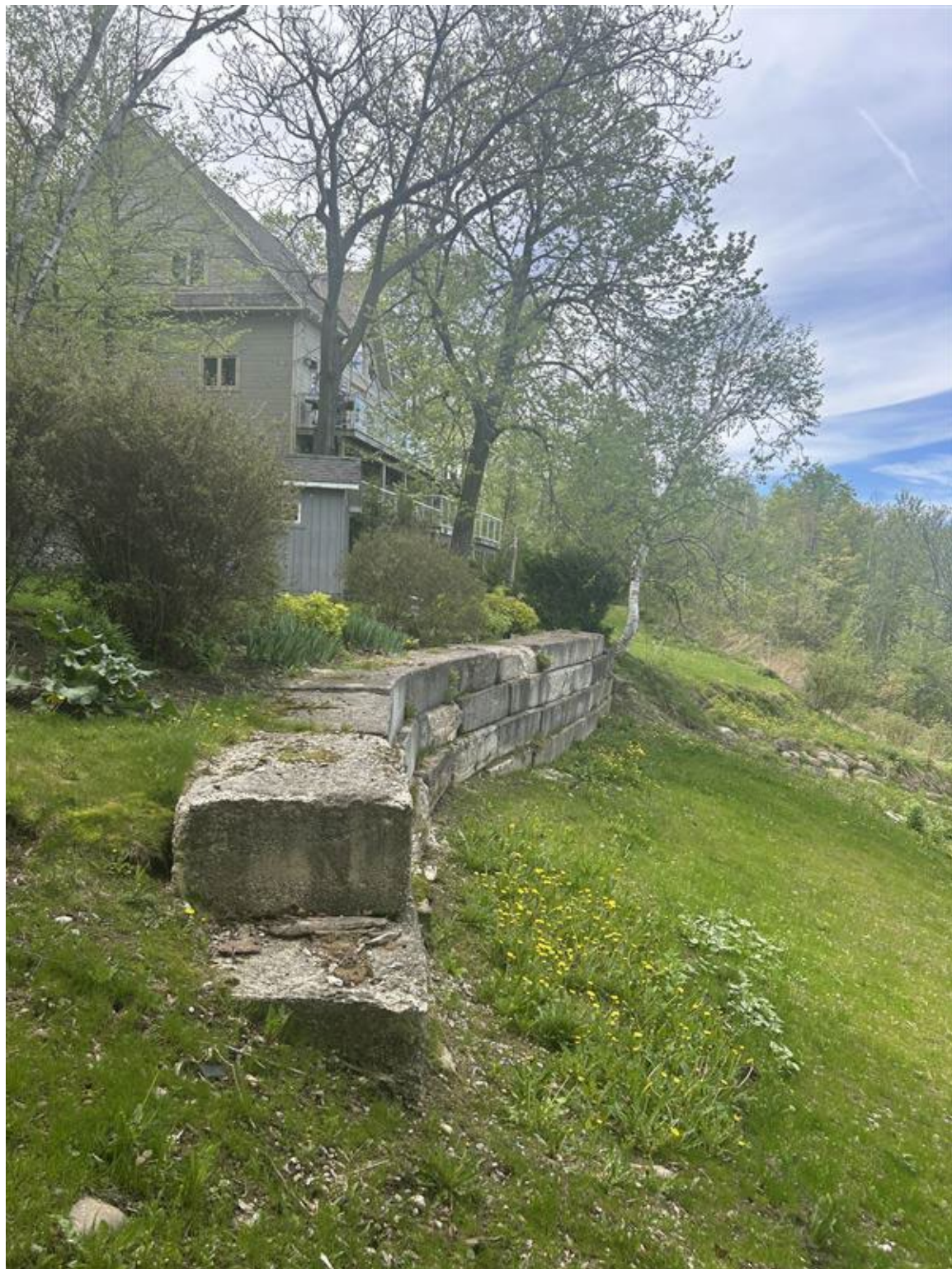
Photograph 3 – View of concrete block retaining wall looking west
