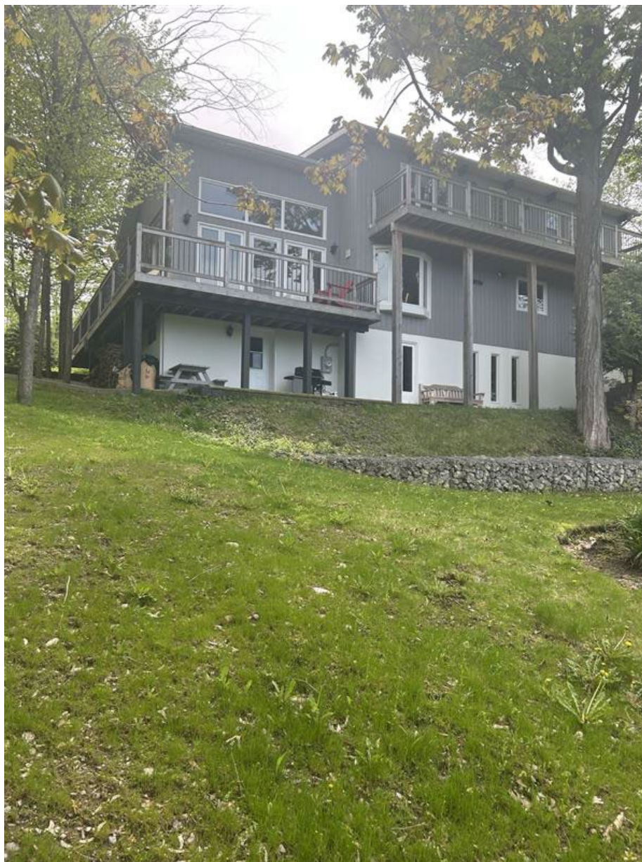
Photograph 1 – View of rear extent of existing dwelling (looking south)
