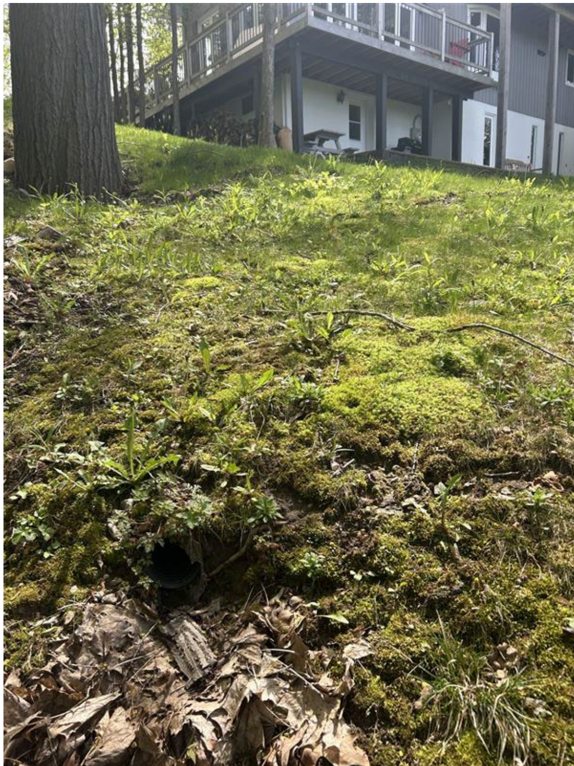
Photograph 7 – View of drainage pipe outflow
