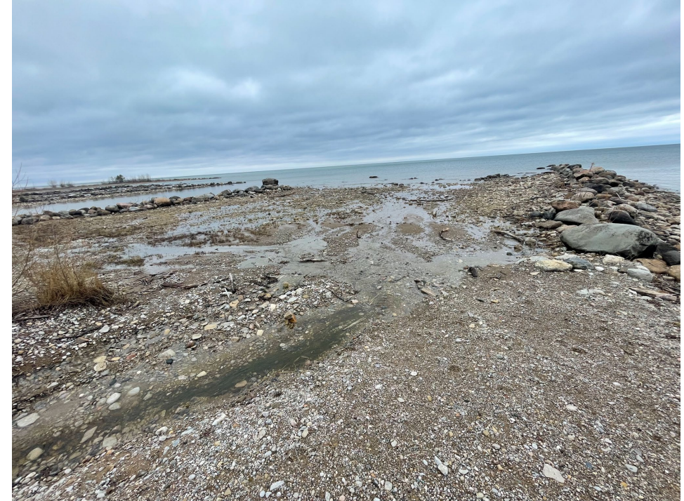
Existing shoreline at Grey St N & Bay St E, prior to construction
