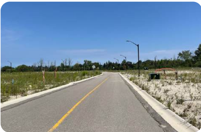
Streets and blocks developed below the ridge
