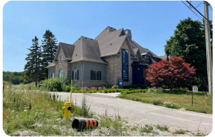
Entrance to Eden Oak Subdivision (under construction)
