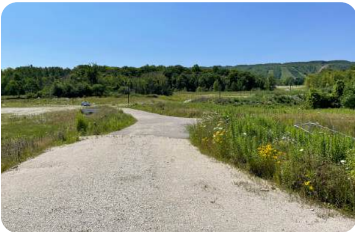
Stormwater pond (north)
