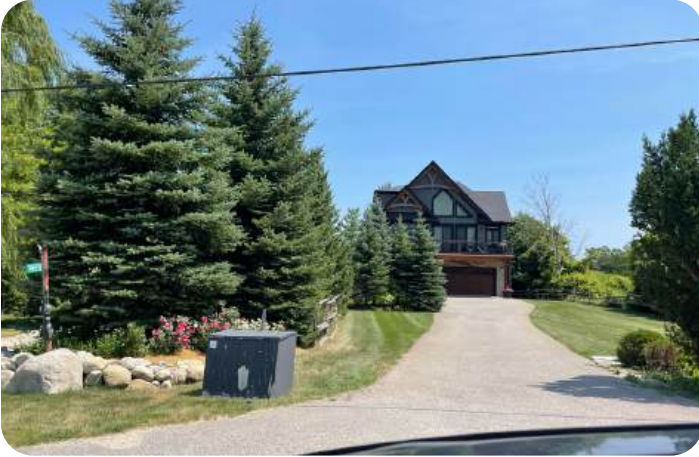
Dwelling fronting on east side of Grey Road 19
