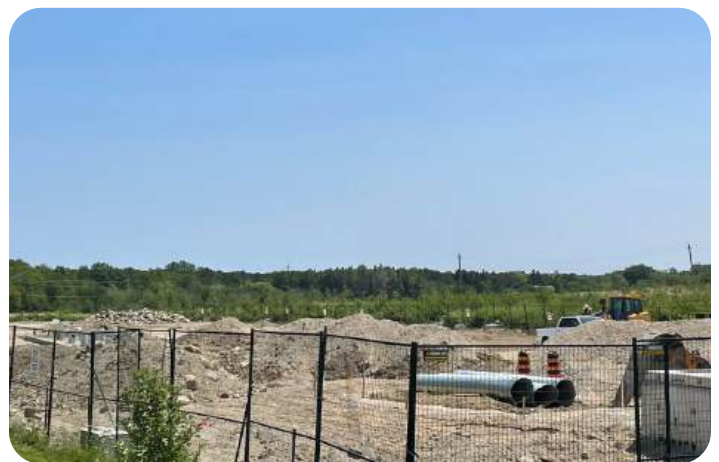
Home Farms Subdivision (under construction)
